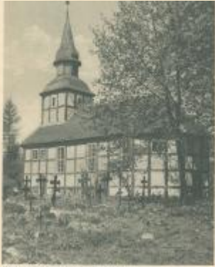
Church in the city of the city of the city of the city of the city of the city of the city of the city of the city
